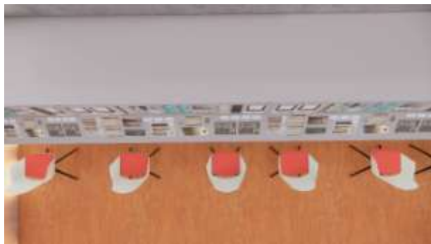
Gambar 4.11 Installation Room Sumber: (Dokumen Pribadi)
